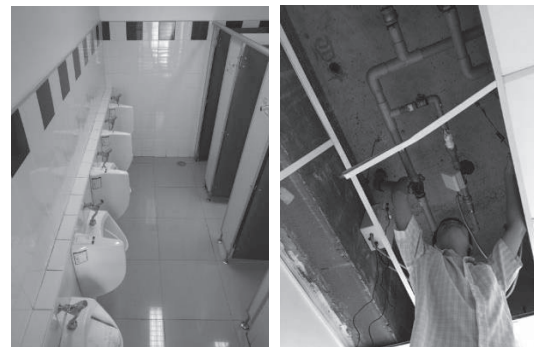
Figure 3 Installation and Testing prototype;
